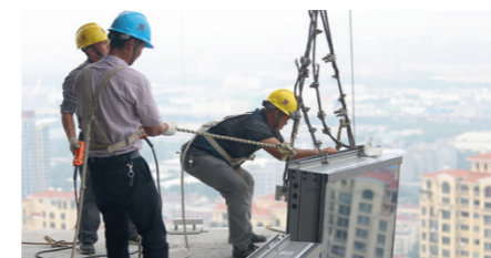
A safe and economic solution for dynamic loads in curtain wall construction.
