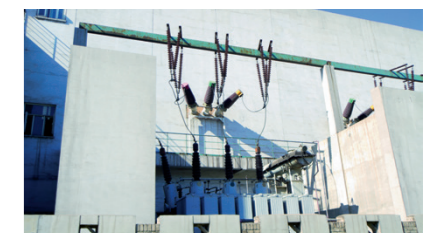
Fixing building appliances.
