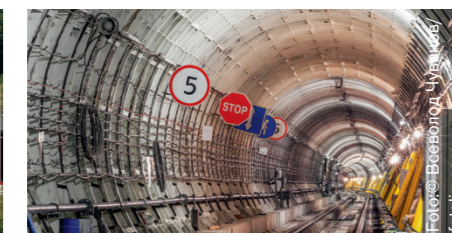
Fixing of signs or supply pipes in tunnel structures.
